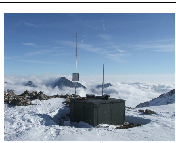
Station sismique SATI - Installation des instruments
