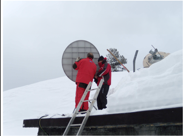
Station sismique RRL – Substitution de la parabole
